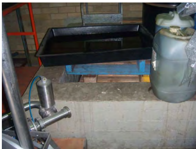
Site Photograph 8: waste oil pit within the eastern portion of the building within Lot 22 DP 620329
