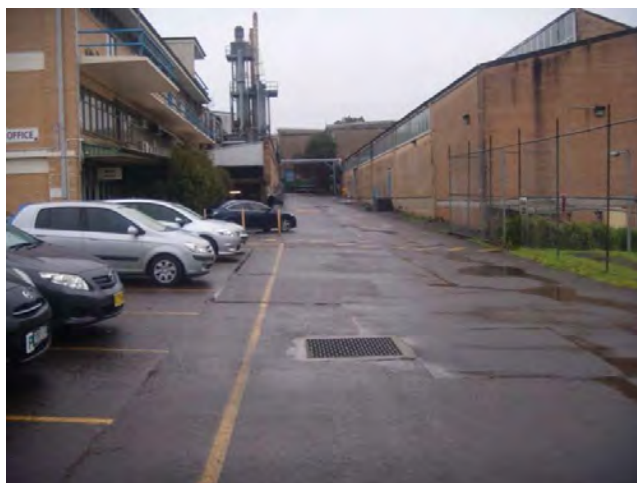
Site Photograph 20: facing west, overlooking the former location of the petrol USTs in Lot 22 DP 620329
