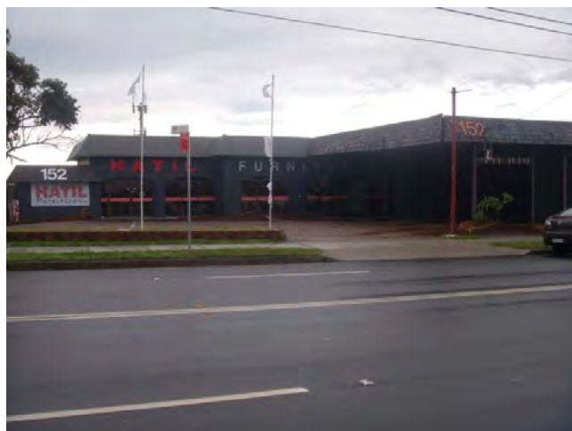
Site Photograph 1: facing southeast, overlooking furniture showroom in Lot 1 DP 405531
