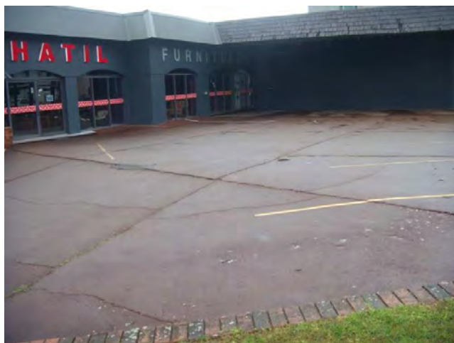
Site Photograph 2: facing southeast, overlooking the bitumen sealed car park within Lot 1 DP 405531
