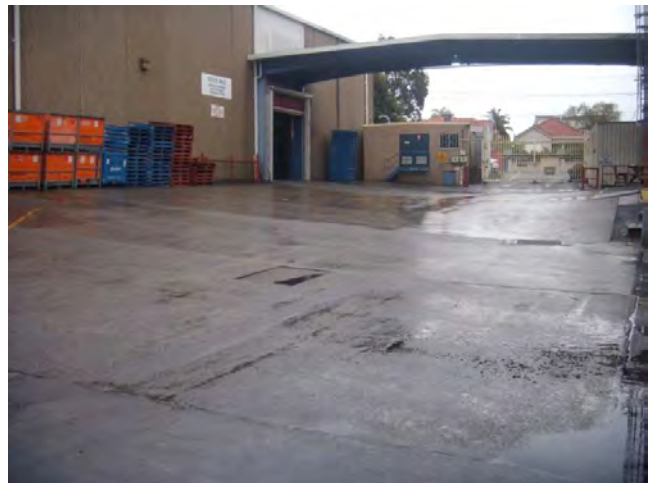
Site Photograph 16: facing west, overlooking the vehicle entrance to Lot 22 DP 620329
