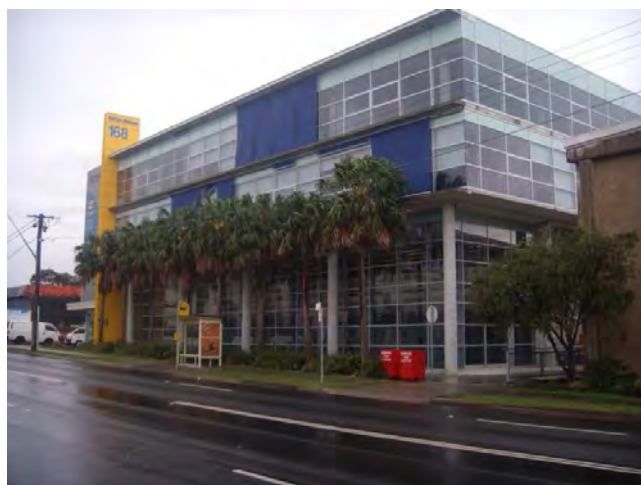
Site Photograph 3: facing northeast, overlooking the new office building within Lot 1 DP 1144981
