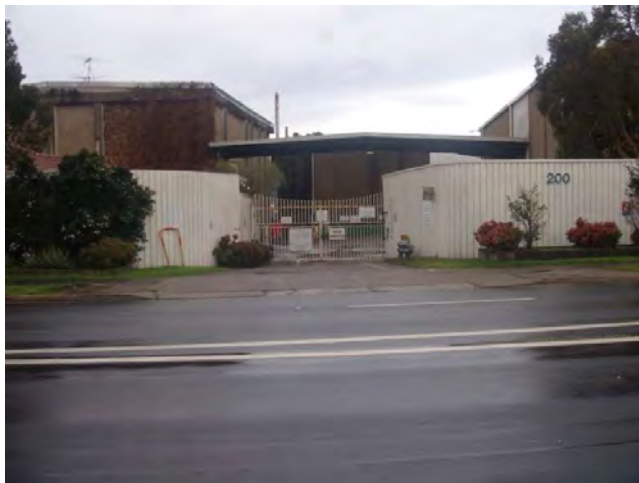
Site Photograph 15: facing east, overlooking the vehicle entrance to Lot 22 DP 620329
